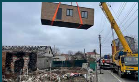
A prefabricated home being lifted into place © DFAT
