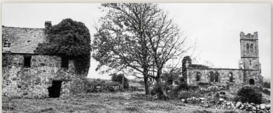
Church of Ireland primary school and church, Ayle.
